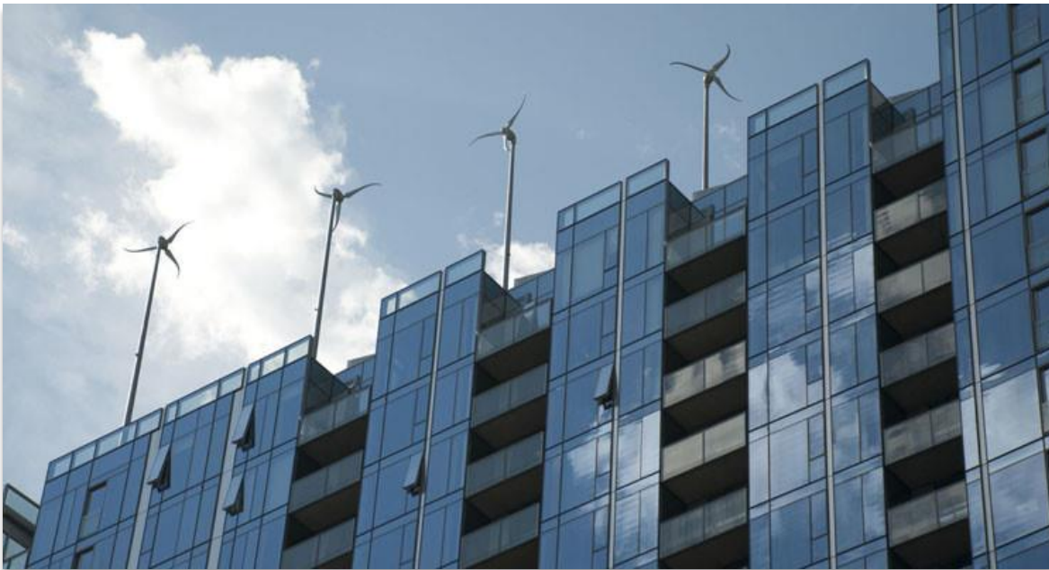
Rooftop Turbines – Portland, Oregon LEED Building
