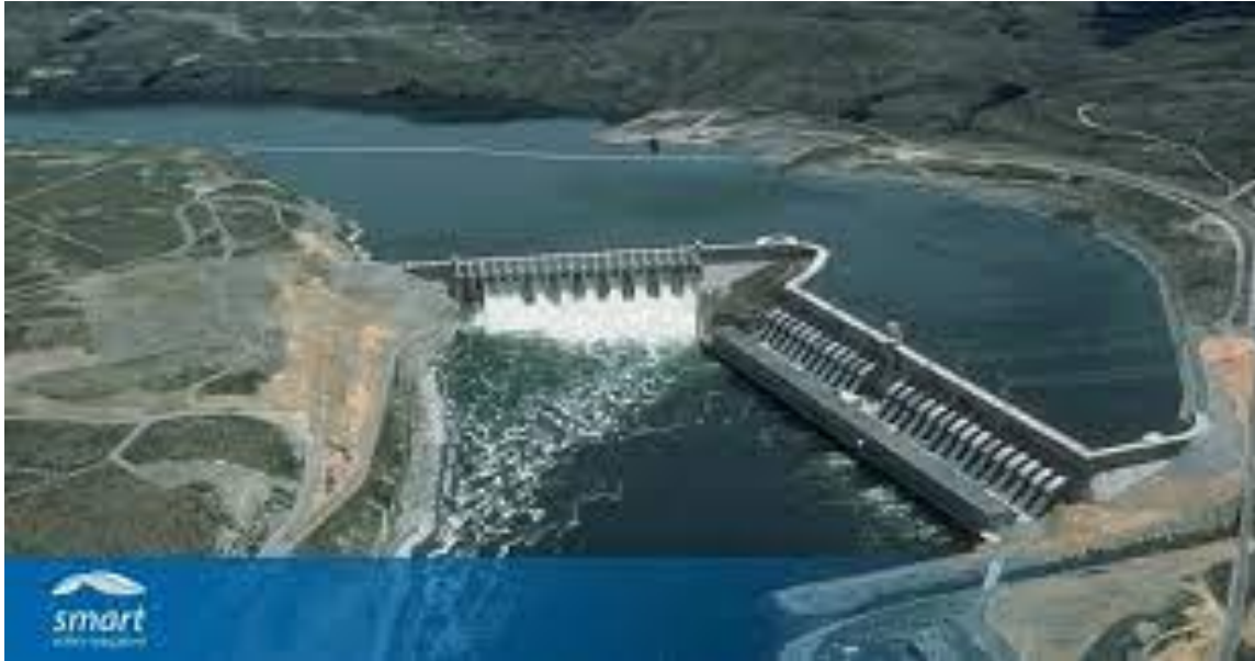
Hydropower Facility. Source: Smart Water
