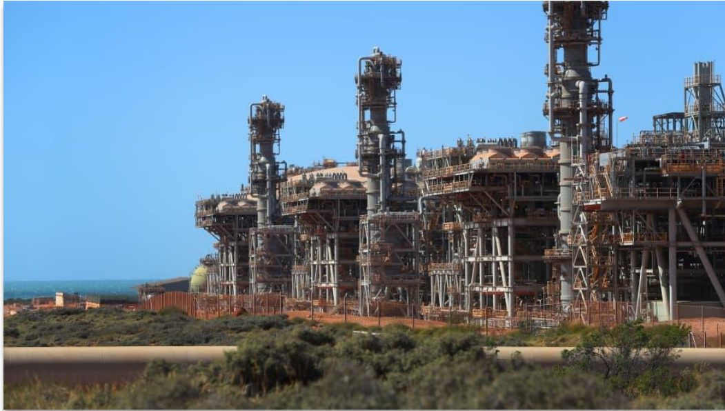
The Gorgon liquefied natural gas (LNG) and carbon capture and storage (CCS) facility, operated by Chevron Corp., on Barrow Island, Australia
